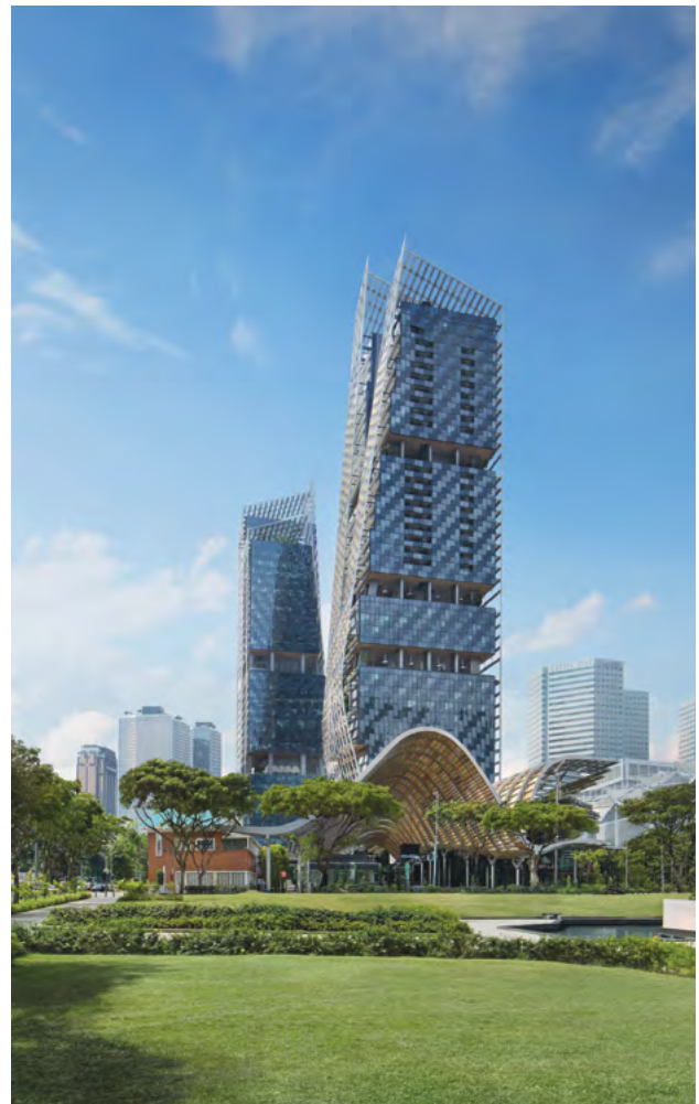
South Beach is a mixed-use development that is strategically located on a part of Beach Road, that borders Singapore's Central Business District.
